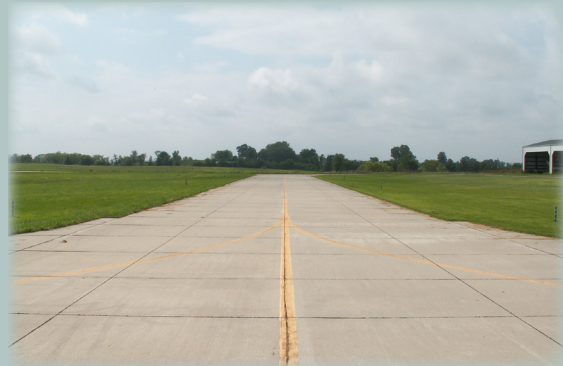
Parallel Taxiway-Looking South
