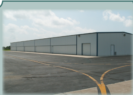
Hangar 200-Looking From Apron
