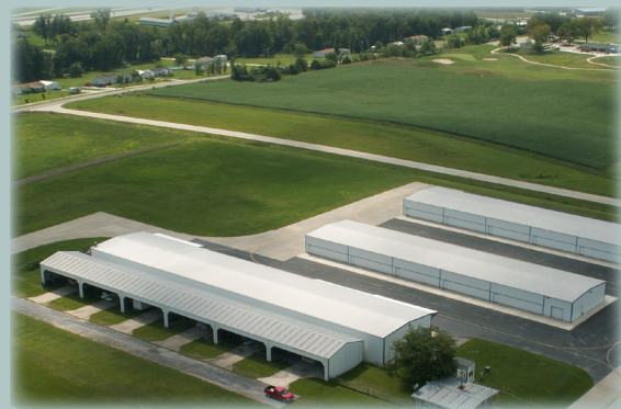
(L-R) Shade Hangars, Hangars 100, 200 and 300
