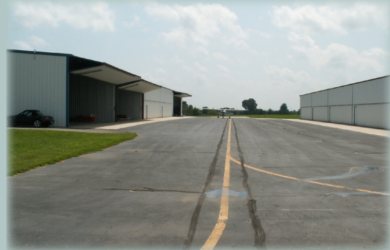
Hangar 100 (L) and T-Hangar 200 (R)
