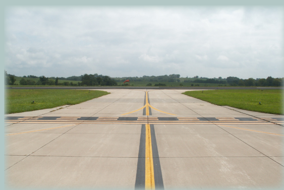
Apron Connector Taxiway
